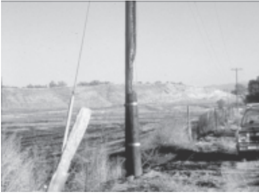
Figure H261A2d-2 Stub pole too short
