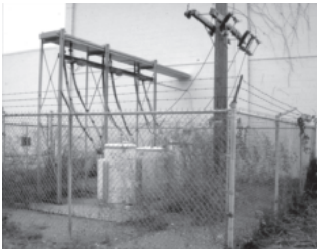
Figure H124C3-3 Padmounted substation not meeting Rules 110A2, 124A1, or 124C3
