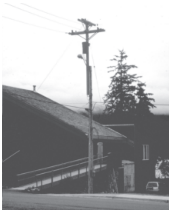
Figure H261A2d-3 Inappropriate side-by-side top pole splice
