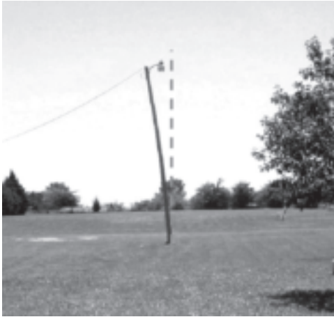
Figure H260-3 Pole deformed by unbalanced service drop tension
