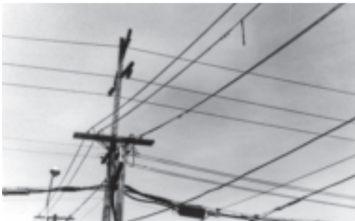
Figure H230-7 Covered conductor with deteriorated covering
