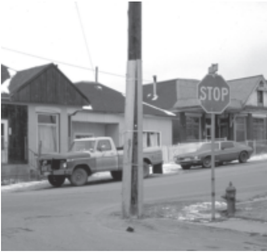
Figure H261A2d-4 Damaged pole with metal splint in location not meeting Rule 231B
