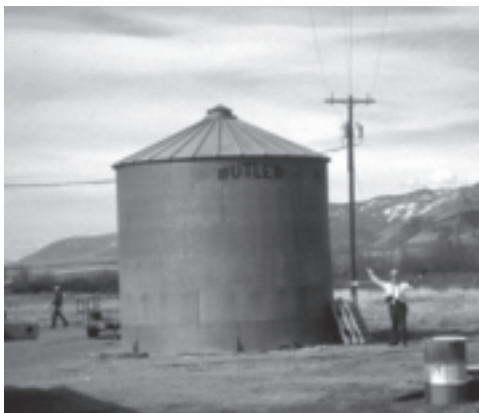
Figure H234F Grain bin clearance less than required by Rule 234F
