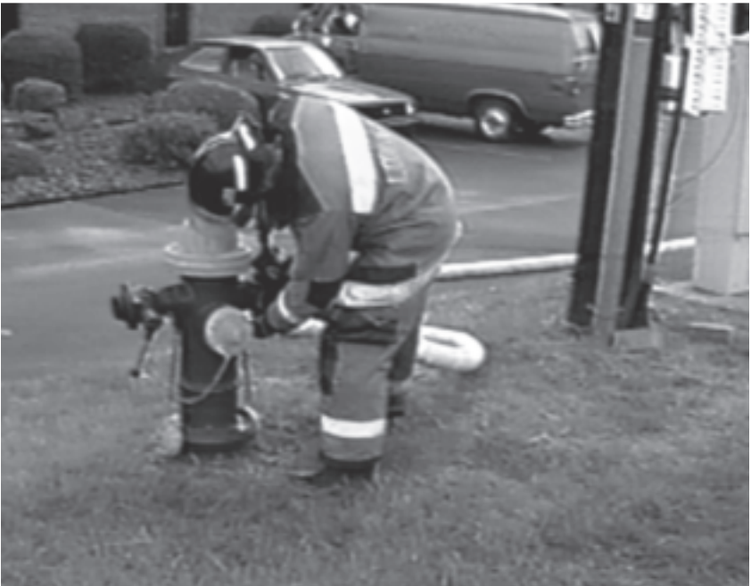
Figure H231-1 Fire hydrant with portable gate valve attached
