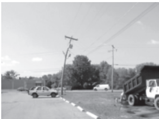
Figure H260-1 Pole overloaded by unguyed angle service drops, and equipment location
